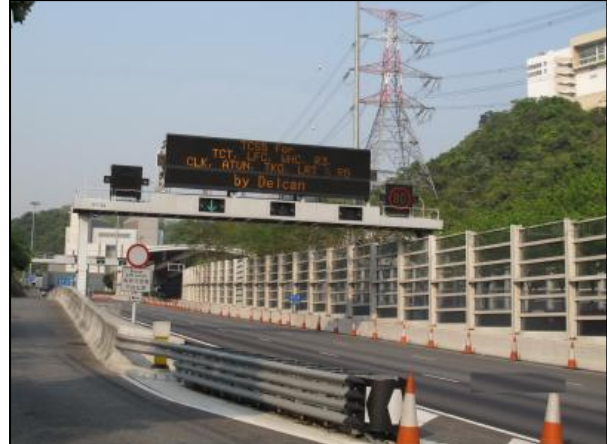
Hong Kong Route 8 Traffic Control
