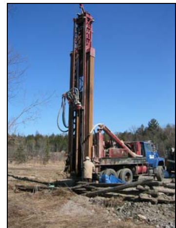
Well drilling rig on site.
