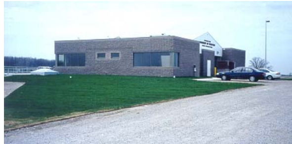
Plympton Wastewater Treatment Plant
